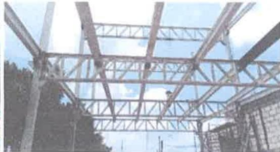
ESTRUTURA DE ACERO, A BASE DE COLUMNAS EN DOBLE MONTEN, ASI COMO VIGAS IPR, Y ESTRUCTURAS EN ARMADURA PARA RECIBIR SISTEMA DE ENTREPISOS.
